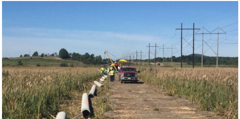
Addison natural gas project construction | VHB
